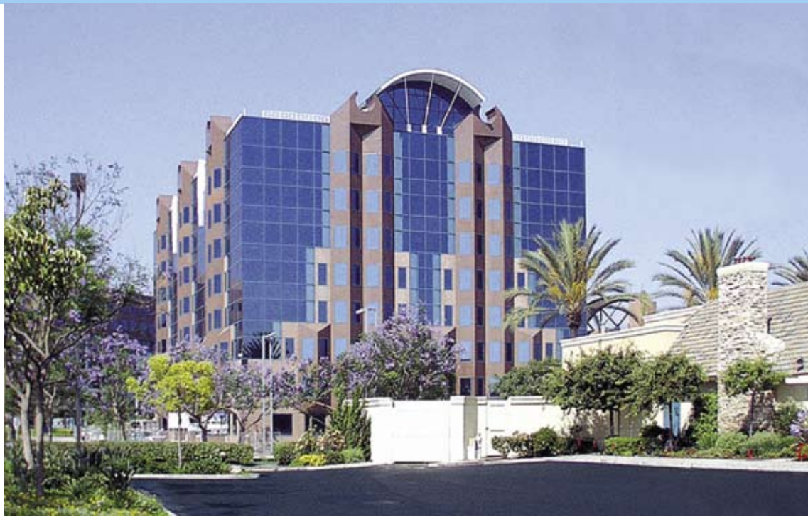
Arden Realty's Cerritos Towne Center (this page) in Cerritos, Calif., and the Governor Executive Centre II (opposite page) in San Diego, are both part of Arden Realty's extensive portfolio
